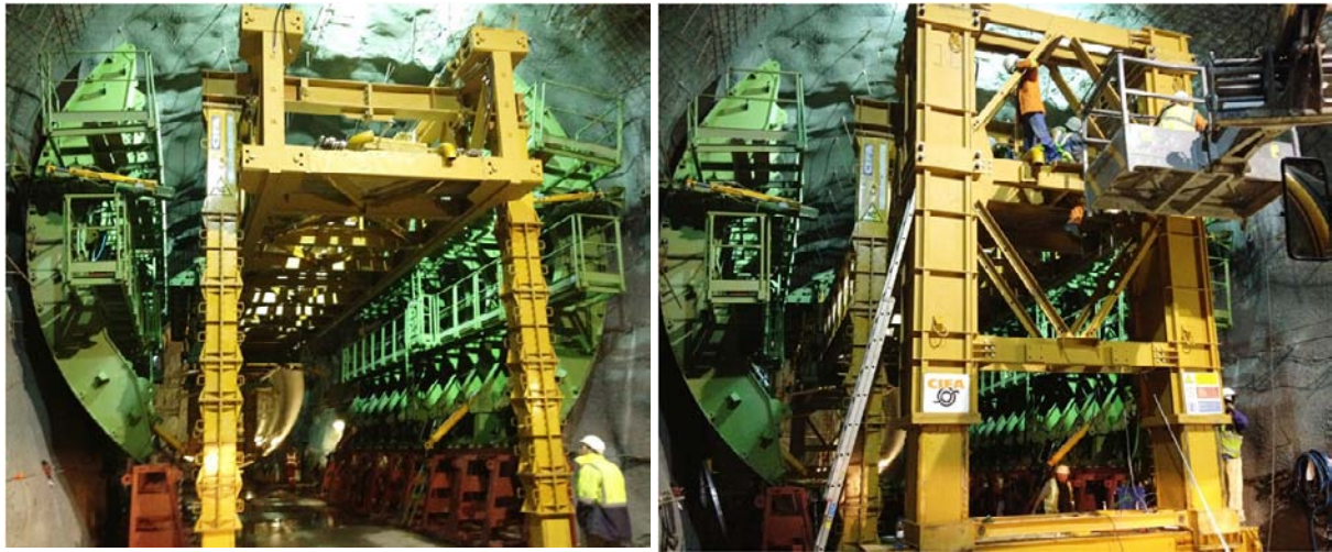
Figure 8. Temporary CIFA lifting mechanisms (left) and final portal structure (right)
