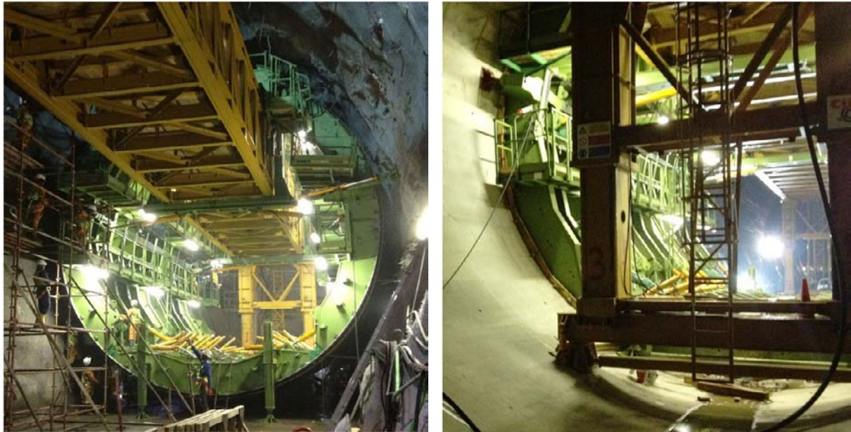
Figure 6. Formwork assembled on the first casting position: front view (left) and rear view (right)
