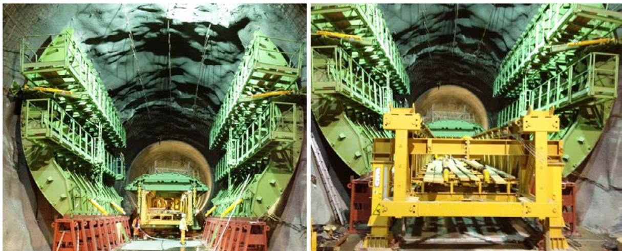
Figure 7. Preassembly of pier and vault forms (left); preassembly of the beam (right)
