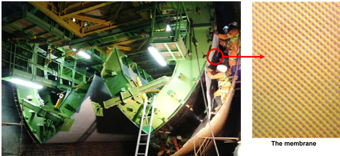
Figure 10. Application of the membrane on CIFA formwork
