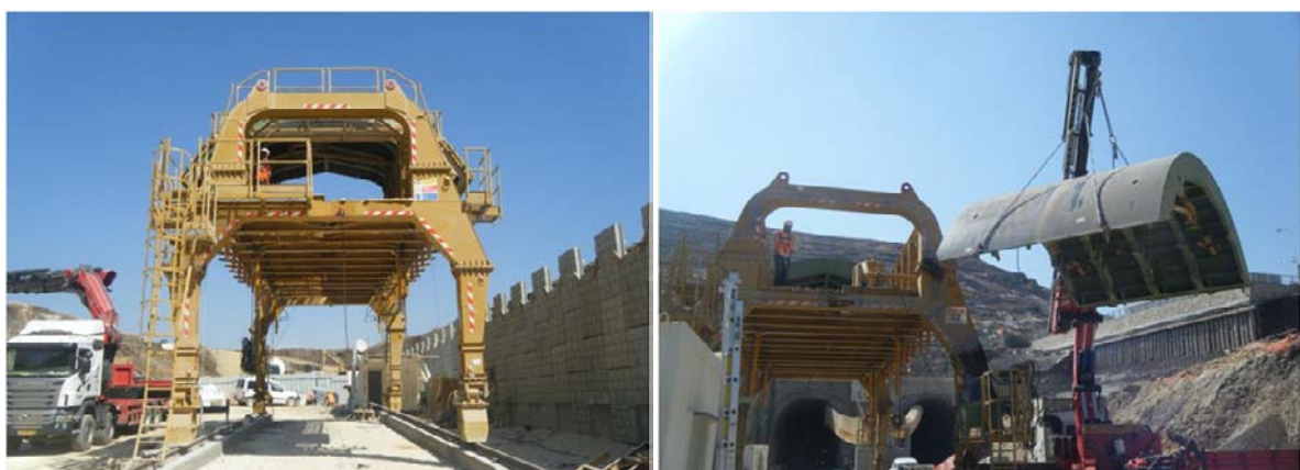
Figure 12. Formwork assembling operation
