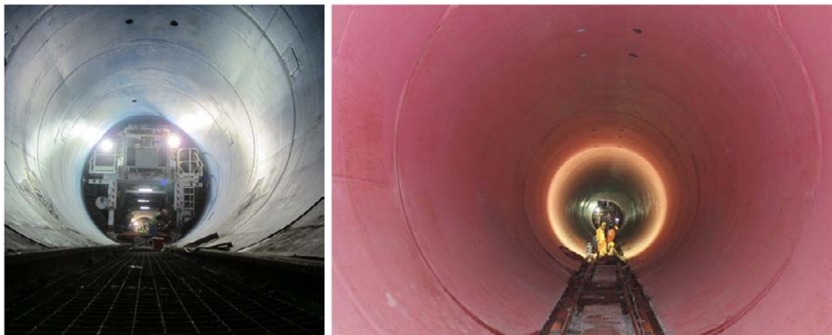
Figure 11. Final Lining with HPDE installed
