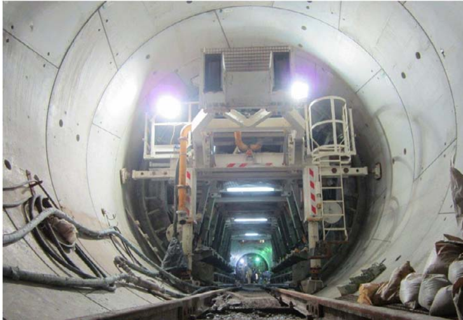
Figure 5. Tunnel Form in curing
