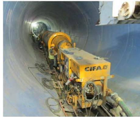
Figure 8. Concrete train during pumping
