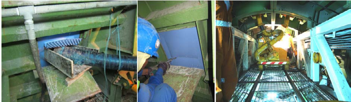
Figure 10. Concrete inlet operation
