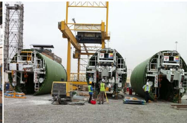
Figure 3. Assembly on site WS 5
