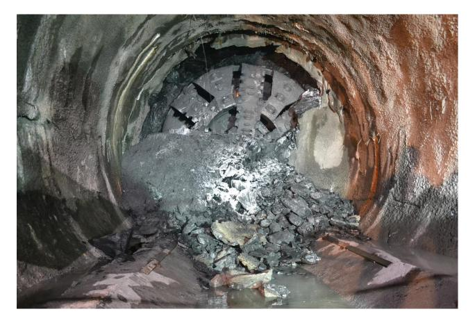
The ground has varied from true mixed ground to soft ground with up to 4 bar EPB face pressure being applied. The machine is now to drag through approximately 200m of station and then will be removed via a 60m deep shaft and relocated to the beginning of the Yenimahalle station and rerun the alignment to complete the section.
