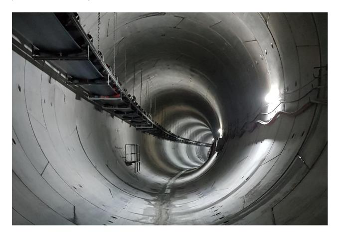
At 7am, on March 03, 2018, one of two TERRATEC 6.56m diameter Earth Pressure Balance Tunnel Boring Machines (EPBMs) employed on the Dudullu-Bostancı Metro Line project, in Istanbul, Turkey, completed an outstanding advance of 19 rings in a single shift. Equating to 26.6m of excavation in just 12-hours, the TBM worked non-stop – alternating between 20-minute mining and ring building cycles – to accomplish a new production record for a TBM of this size and class in Istanbul.
