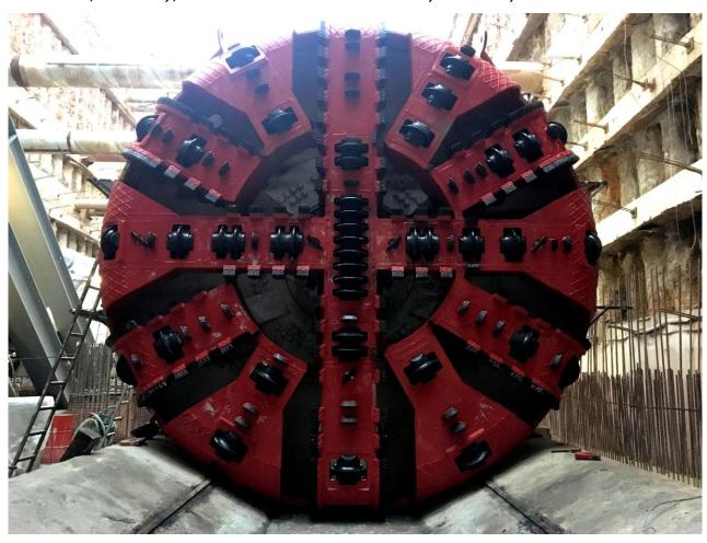
Two TERRATEC 6.56m diameter Earth Pressure Balance (EPB) Tunnel Boring Machines are making good progress on the latest expansion of Istanbul's Metro system, with both machines now fully up and running and achieving good advance rates for the project.
