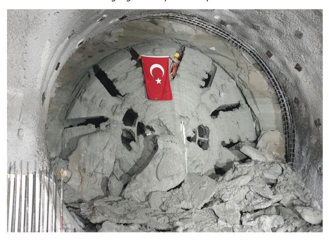
TERRATEC is pleased to announce that the first of four new 6.56m diameter Earth Pressure Balance Tunnel Boring Machines (EPBMs) currently working on the Ümraniye-Ataşehir-Göztepe (UAG) Metro line – which is being constructed by the Gulermak, Nurol & Makyol JV – successfully completed its first intermediate breakthrough on 20 May, into Atasehir Station.
