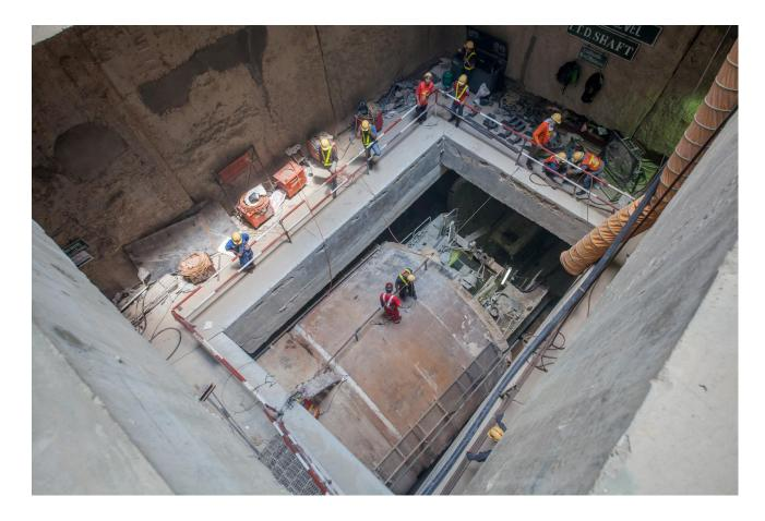
The EPBM had to bore through as many as eight (8) diaphragm walls, as well as several obstacles such building foundations. This was expected at the beginning of the project and for this purpose, TERRATEC selected a unique CutterHead design with conical shape to overcome those smoothly without disrupting the soil around.
