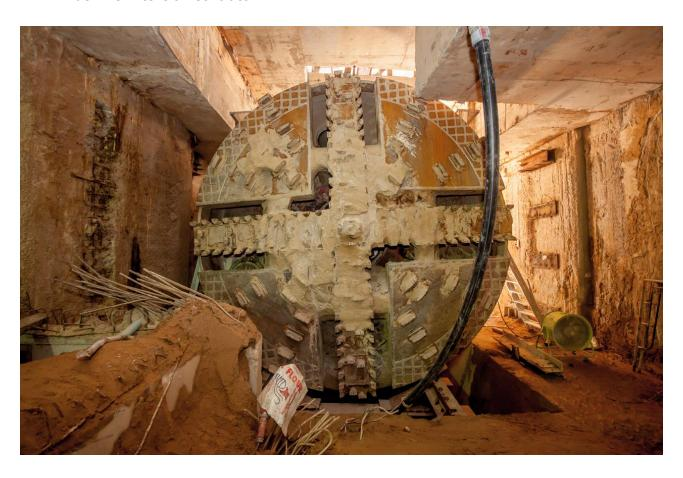
Contractor, Italian-Thai Development PLC, used the machine to bore this 2,800 meter long alignment in one go, crossing two unexcavated stations and one ventilation shaft on its way. Next drive along the East Bound of the line, will have the stations completed as the TBM arrives, so it will be dragged through those.
