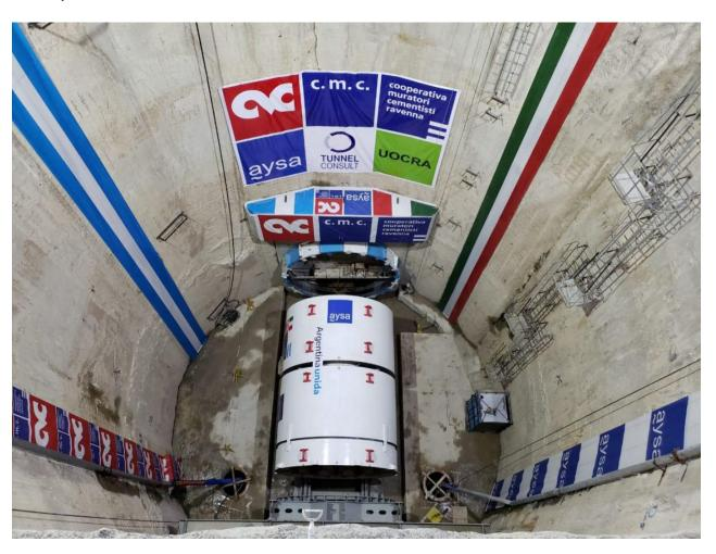
TERRATEC is pleased to announce that the first of two 4.66m diameter Earth Pressure Balance Tunnel Boring Machines (EPBMs) that will be used to excavate the Río Subterráneo a Lomas tunnel is currently being assembled, in Buenos Aires, Argentina.
